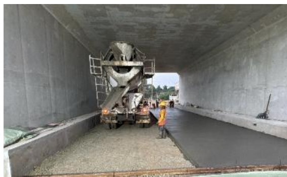
Gambar 7. Pekerjaan Lean Concrete
